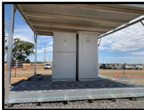
Figure 14 Typical HV switchboard and platform (Source: AC Energy)
